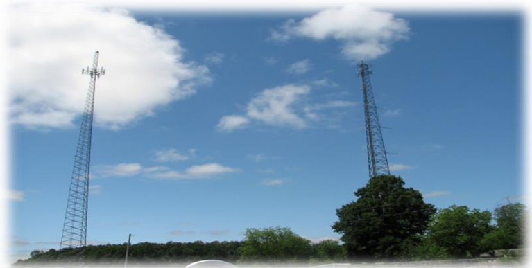
Two monitoring towers in Arkansas used to collect data on wind speeds. Credit: AWS Truepower, LLC
