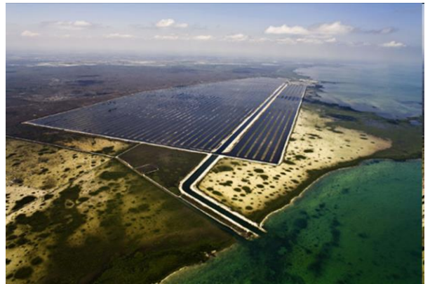
Cooling canal system at FPL's Turkey Point which recent study shows are contaminating the Biscayne aquifer and National Park.
