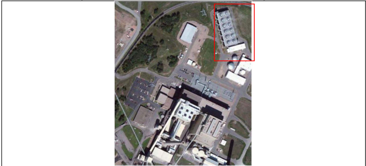
Figure 2. 12-Cell Back-to-Back Mechanical Draft Cooling Tower 7
