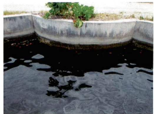
Photo 2-1. Hardened shoreline of barge canal
