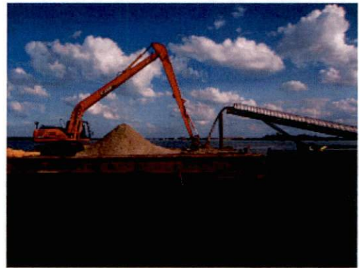
Photo 3-2. Fill conveyor loading placement barge
