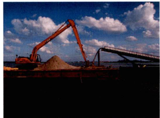
Photo 3-3. Fill conveyor loading placement barge
