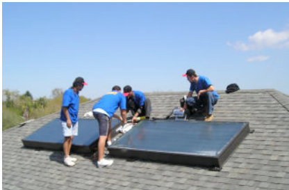
Solar Source technicians installing a domestic hot water unit (DHW) on a home in Seminole, FL. Solar DHW can reduce a power bill in a single family home by up to 40%.
