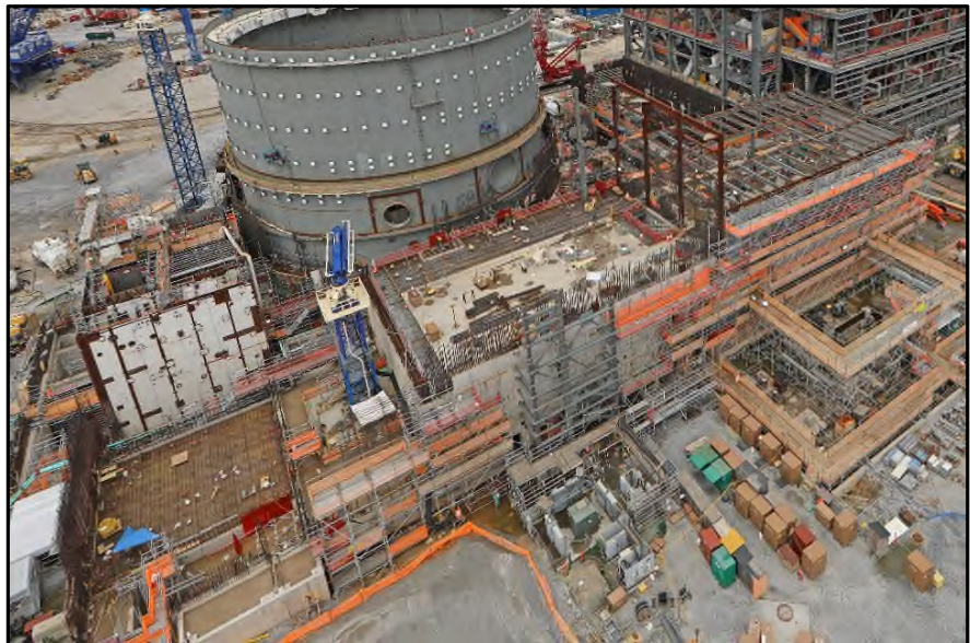
Photo 5 – Unit 3 Annex Building
