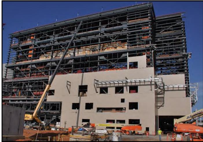
Photo 4 – Unit 3 Turbine Building Exterior
