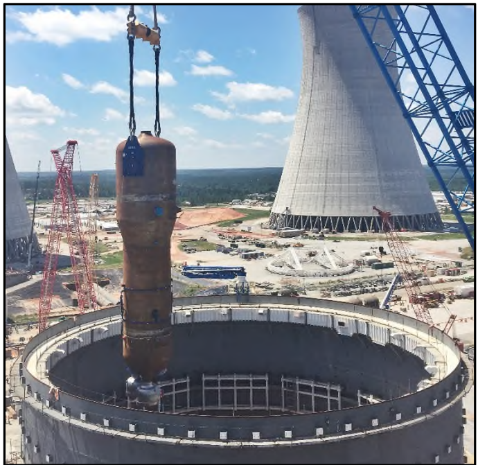
Photo 2 – Setting of Unit 3 Steam Generator
