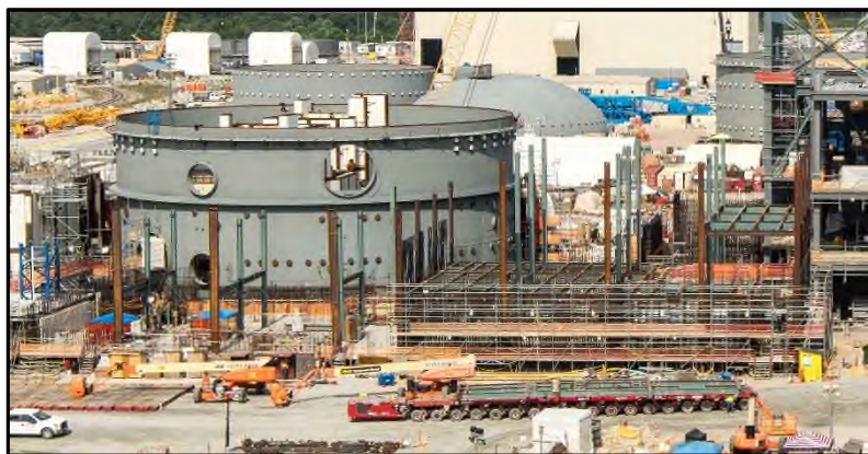
Photo 8 – Unit 4 Annex building
