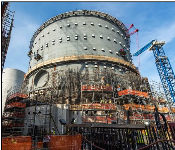
Photo 3 – Unit 3 Containment Vessel and Shield
