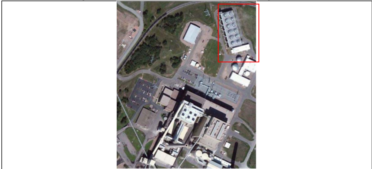
Figure 2. 12-Cell Back-to-Back Mechanical Draft Cooling Tower 7
