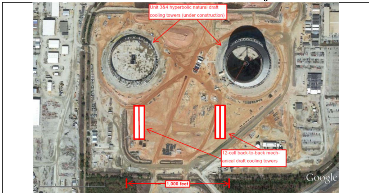
Figure 3. Hyperbolic Natural Draft Cooling Towers Under Construction at Vogtle Units 3 and 4 and Possible Locations for 12-Cell Back-to-Back Wet Cooling Towers 8
