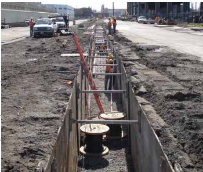
Burying power lines makes them less vulnerable to extreme weather and can help prevent outages, but that step is also expensive. PSE&G—a New Jersey utility hit hard by hurricanes Sandy and Irene—is proposing to spend almost $4 billion over the next 10 years on these types of hardening measures.
