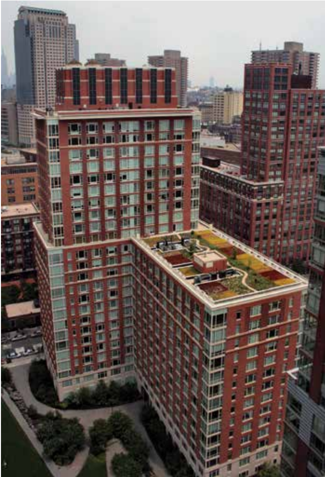
Green roofs—such as this one in New York City—help keep buildings cool and reduce the urban heat-island effect, cutting the amount of electricity used for cooling.
