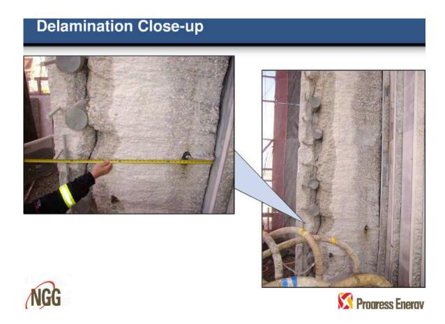
Not only did this 60-foot long crack occur after Progress Energy and B&W had conducted a thorough engineering analysis that was approved by the NRC, more importantly, a second crack developed in 2011 while Progress Energy was still attempting to repair the first crack Crystal River. Once again, the recovery process was thoroughly re-engineered and approved by the NRC and yet it failed for a second time. The net effect of both of these two Crystal River cracks is that a 5-year repair process
