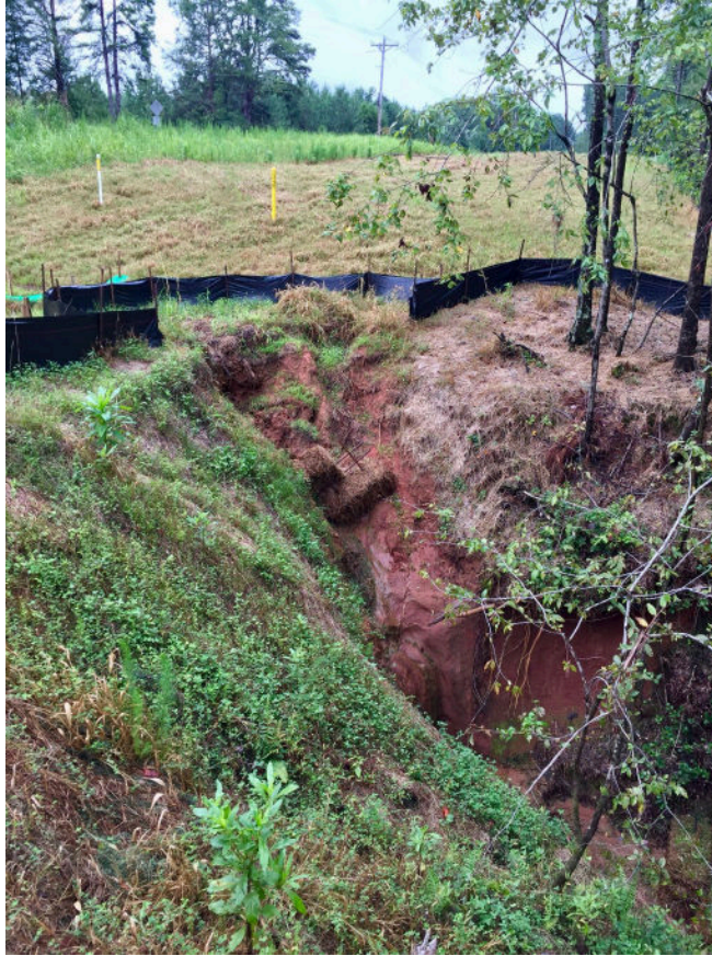
Gully encroachment along the Dominion (now Carolina Gas Transmission/Berkshire Hathaway) Transco to Charleston pipeline project in Spartanburg County, SC (photo/Shelley Robbins)
