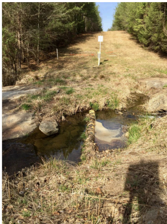
Exposed pipeline in the Upstate of South Carolina (photo/Shelley Robbins)
