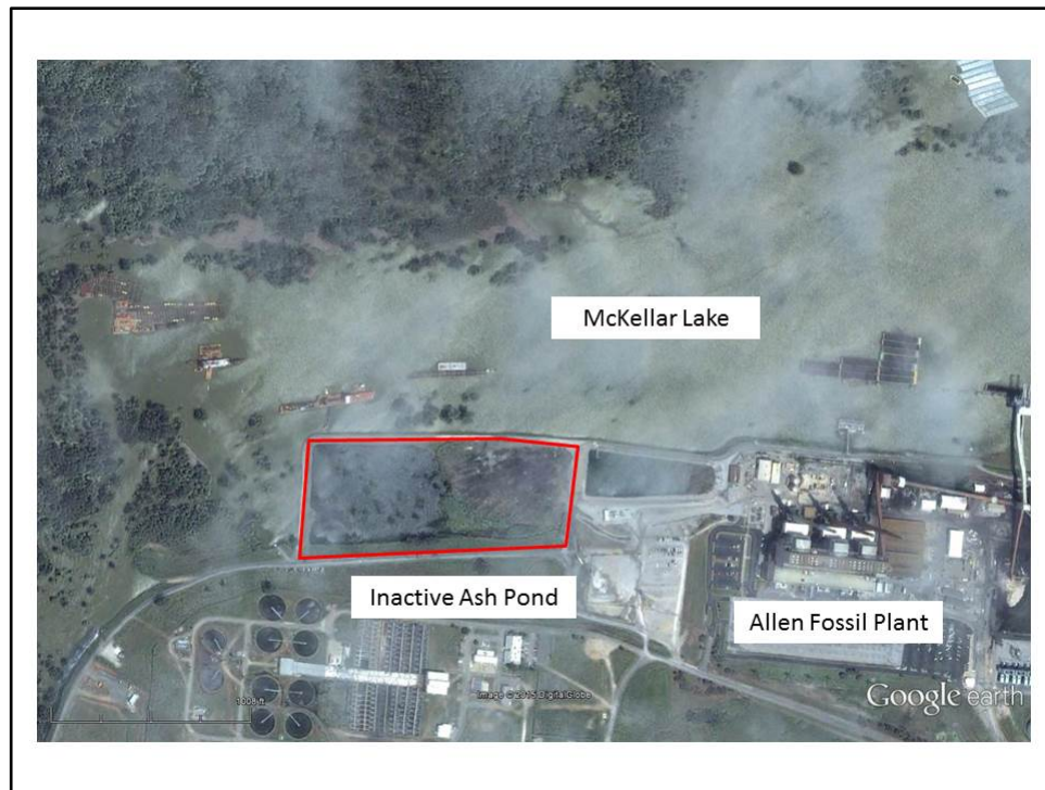
Figure 1: Inactive Ash Pond at the Allen Fossil Plant, May 9, 2011. 17
