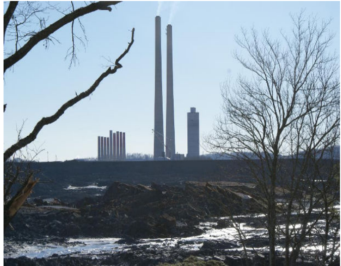
The December, 2008 coal ash spill in Harriman, TN with TVA's Kingston coal plant in the background.
